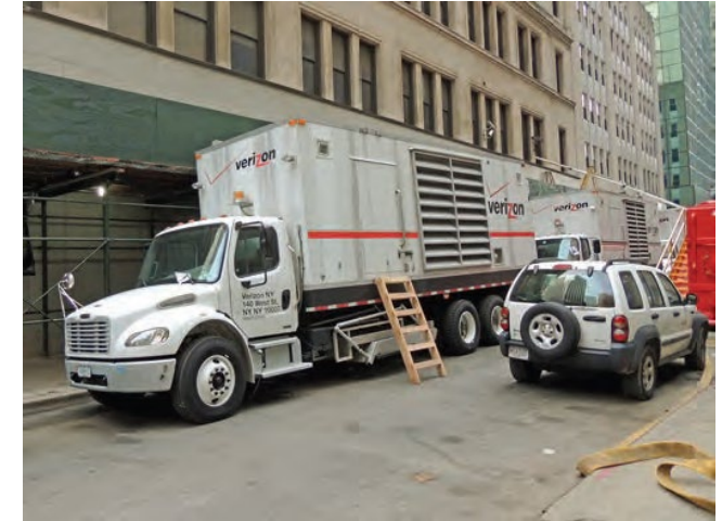
Generators to replace failed basement generators at a data center
