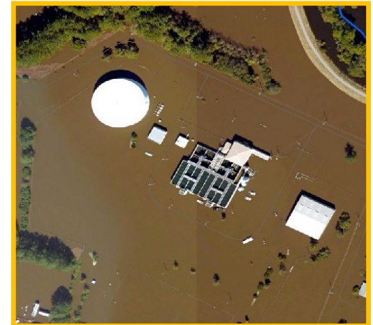
Lumberton, NC Water Treatment Plant Inundation from Hurricane Matthew in 2016
