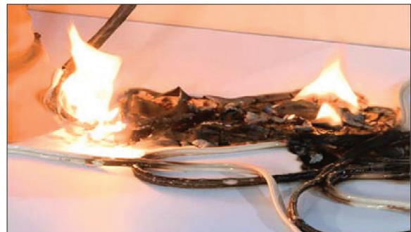
FIG. 22: Overheated Counterfeit Extension Cord.
