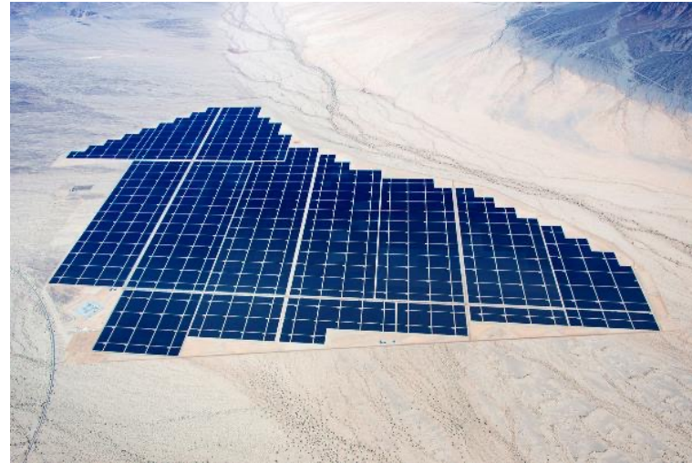
550 MW CdTe solar farm in the Mojave desert
